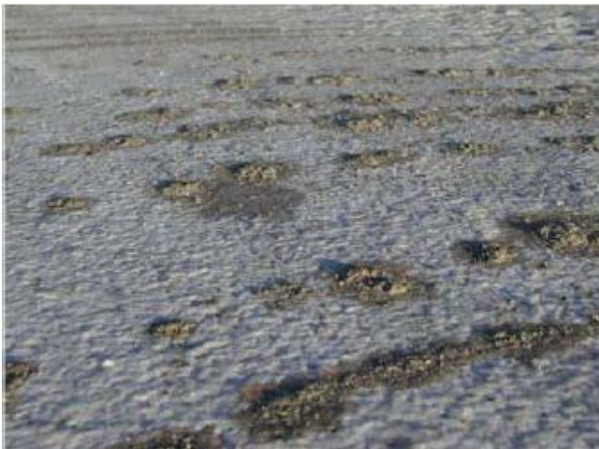
Figure 2.9: Sand Prewet with Hot Water on a Roadway (Transportation Research Circular, 2004)
